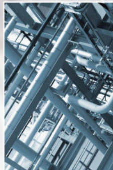
Heating equipment inspection
